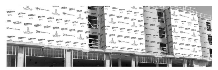
Ensuring the compatibility of sealants, adhesives, and primers with DRYline water-resistive barriers (DRYline WRBs) and DRYline Self-Adhering Flashing Products, such as building wraps and self-adhering flashings, is important for the long-term performance and durability of a wall assembly. The sealant, adhesive, or primer should be chemically compatible with adjacent DRYline building envelope products used within a wall assembly.
